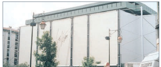
The first textile façade for a multi-story garage in Avignon, France (installed in 1994)
